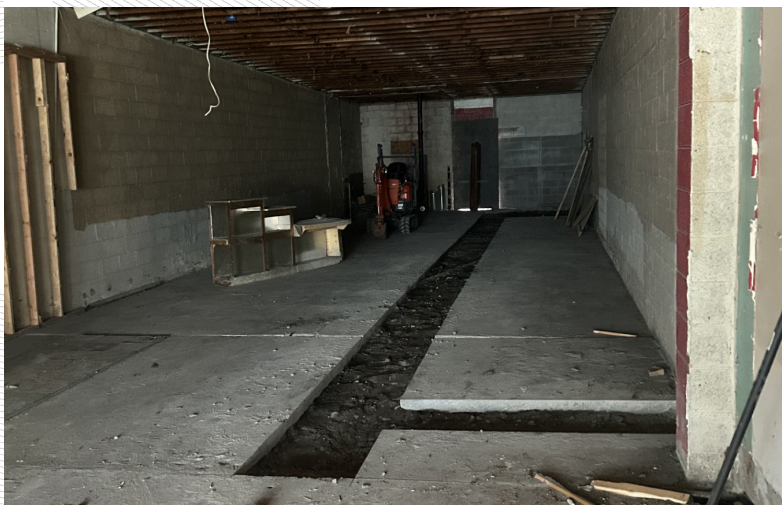
An empty building before reconstruction of a space for mixed use in Mt. Pleasant.
